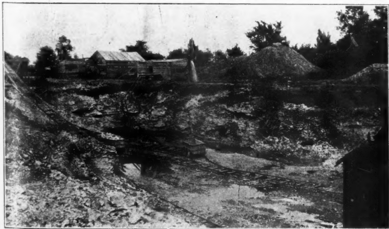
View of Quarry Showing Pumping
